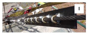
The required number of wire rope grips can now be fitted to the rope using a Ropetech 'Alignment
