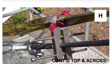
Before the grips can be fitted it is necessary to close the 'live' and 'dead' or tail part of the wire rope around the thimble; in this case the thimble is on the end of a rigging screw.
